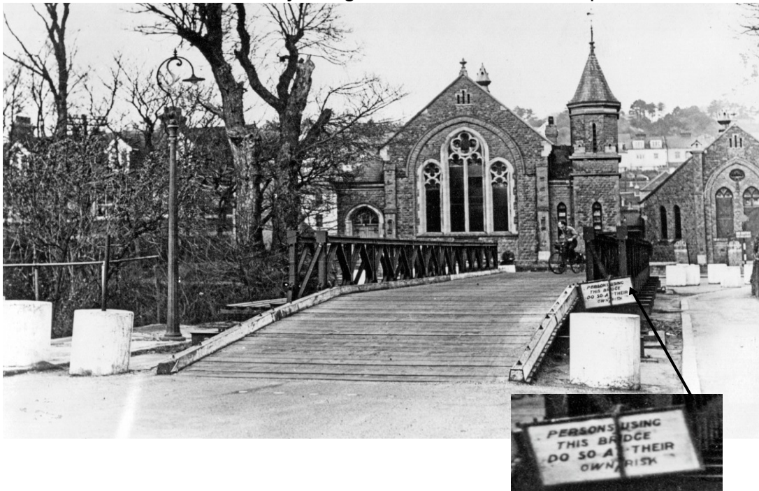
View of Bailey Bridge from Stade St to Rampart Road
