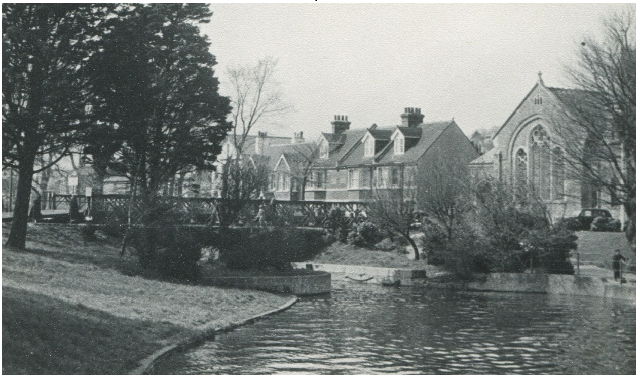
The Bailey Bridge, looking towards Wesleyan Methodist chapel and Rampart Road.
