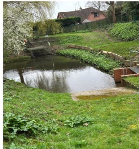
Turnpike Hill flood defences
